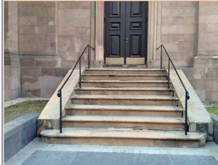
Photograph of existing south stairs before removal. Note step at door and shallow landing
