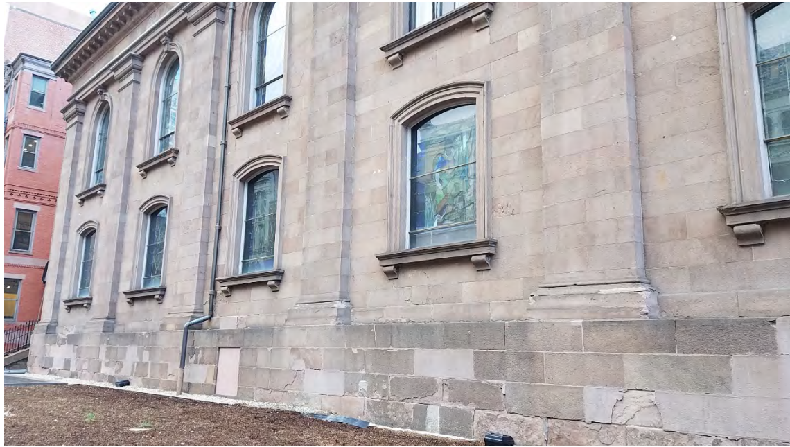
South elevation brownstone water table
