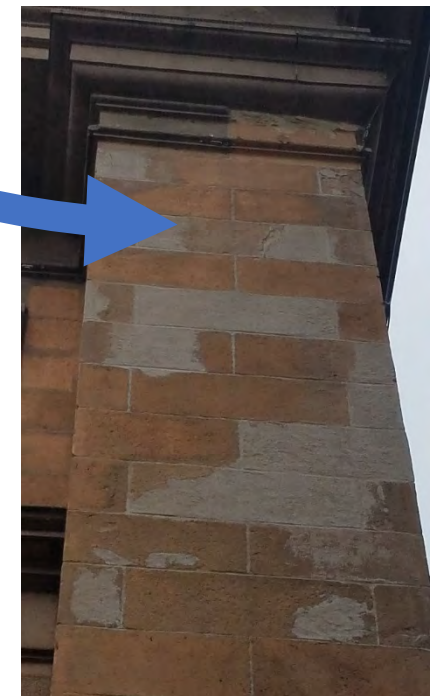
Install harvested stone at pilasters
