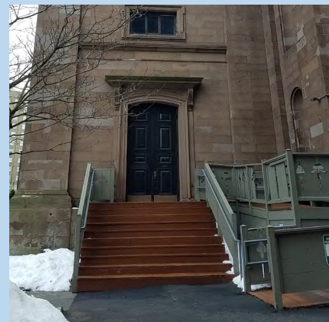
Existing north wood stairs constructed on top of original stone stairs
