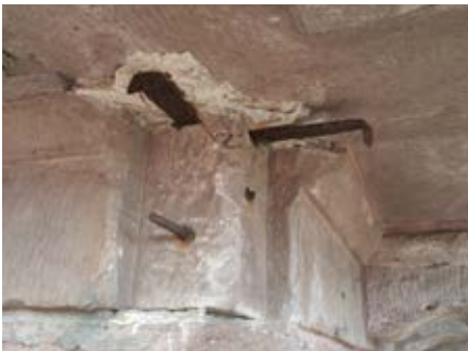
Lost corner modillions leaving ferrous anchors bare and vulnerable to corrosion
