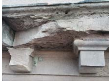
Loss of essential architectural lines and hazardous deterioration over entry
