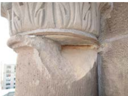
Void after removing a ten-pound piece of unsecured stone perched directly over the entrance
