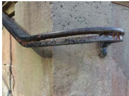
Deteriorating wrought iron handrails at entrance stairway
