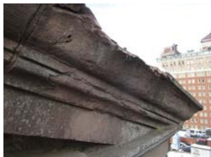
Leading edges of detail with extreme deterioration, friable stone, moisture damage, and biological growth
