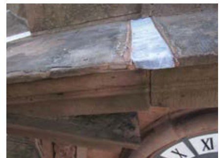
Skyward facing joints that have suffered failed treatments and remain open to moisture incursion
