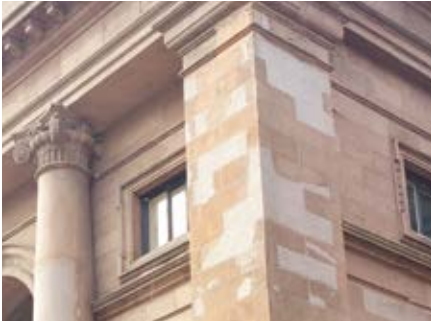
Unsightly and failing patches marring the uniform appearance of the natural stone
