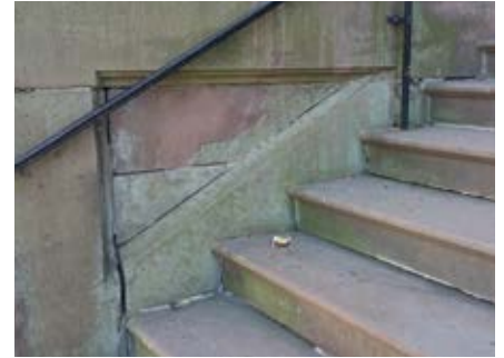
Failing cheek walls on entry stairs with joints open to moisture incursion
